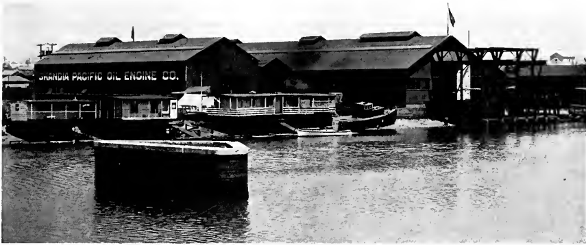
The waterfront at the Skandia Pacific Oil Engine Company's plant, showing extension of overhead crane tracks for unloading and loading supplies and installing machinery in vessels.
